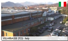
VILLARBASSE (TO) - Italy
