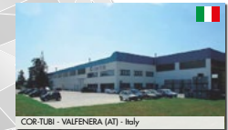
COR-TUBI - VALFENERA (AT) - Italy
